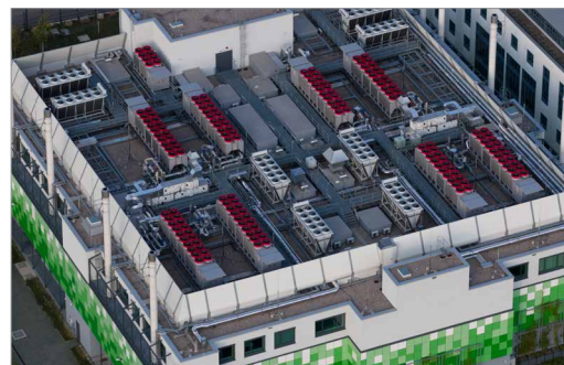
Data centre rooftop cooling system installation
